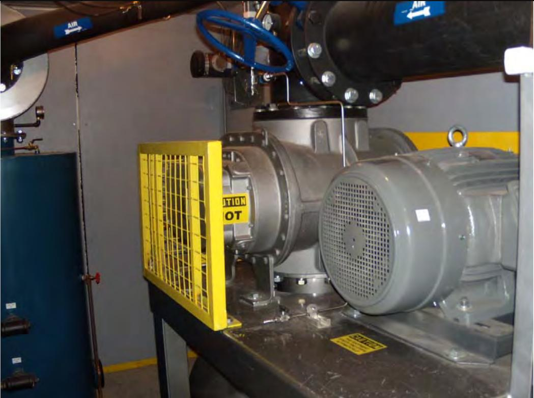
A photograph of a large industrial blower unit. The unit is primarily grey and is mounted on a dark metal base. A prominent yellow safety cage with a grid pattern is positioned in front of the blower. A blue handwheel is visible on top of the unit. The background shows a grey wall with some pipes and a blue door. |                                       |
