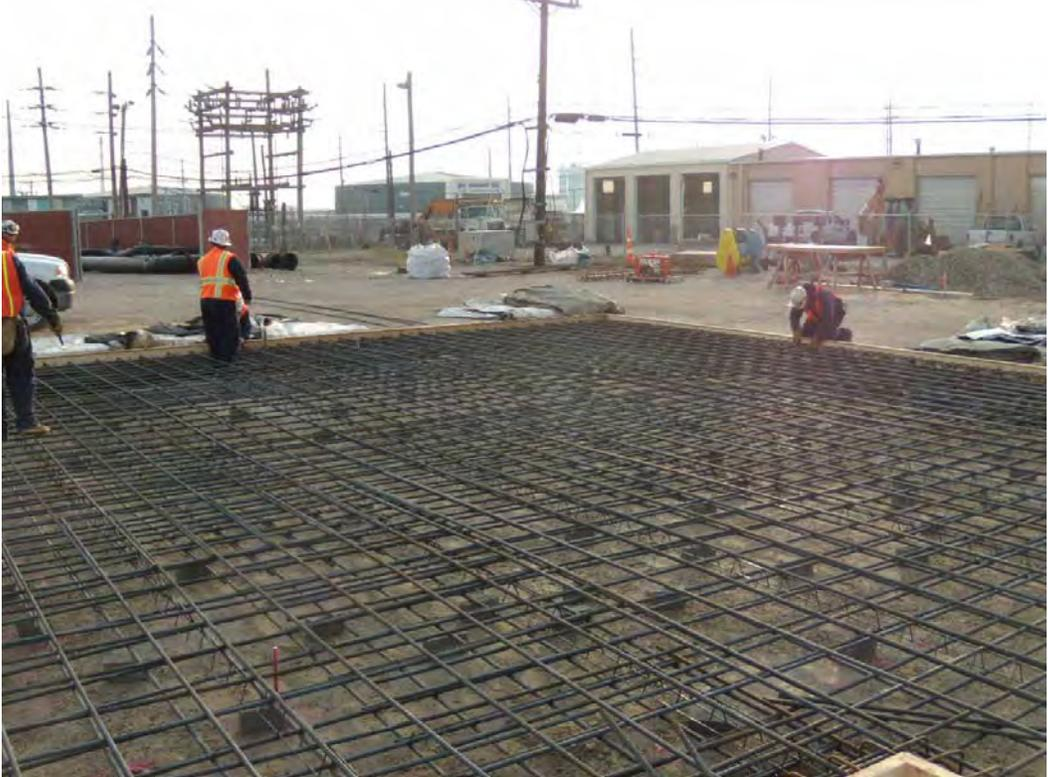
A close-up photograph of a construction site. The foreground is dominated by a dense grid of steel rebar laid out on a concrete slab. Several workers in safety vests and hard hats are visible in the background, some appearing to be working on the rebar. In the far background, there are utility poles, a building with a red roof, and other construction materials. |  |
